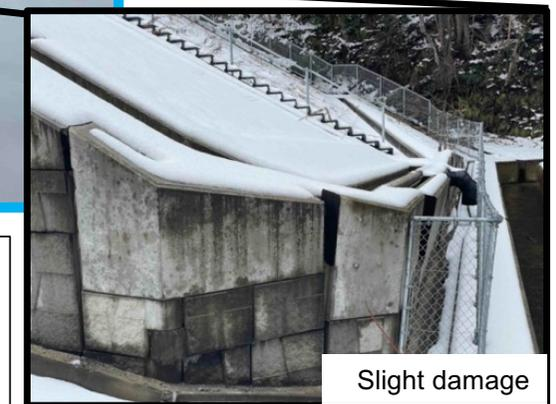
No collapse or major damage was observed in this embankment. Well-maintained drainage possibly helped in quick dissipation of excess pore water pressure created during excessive shaking.
