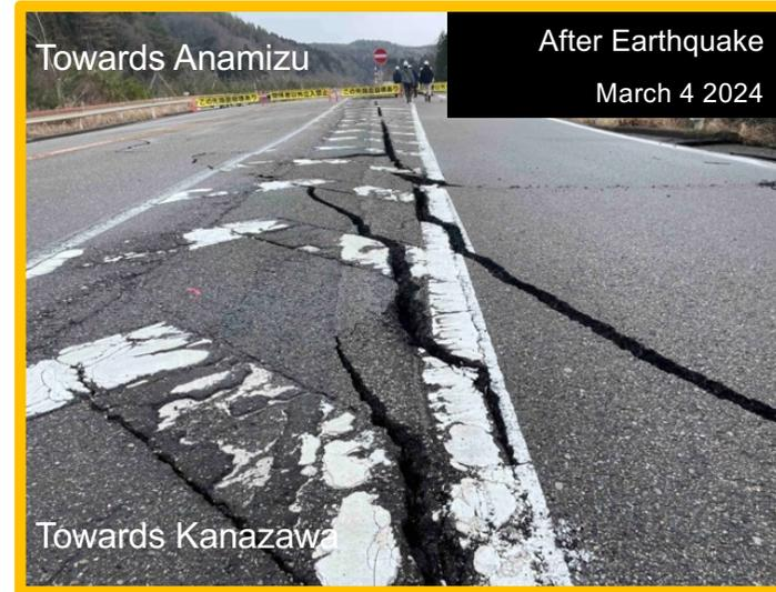
Large cracks were seen on the road surface in the yellow zone. There was no evidence of the embankment collapse.
