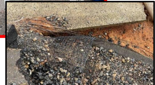
Exposed geotextile from after 2007 EQ retrofit
